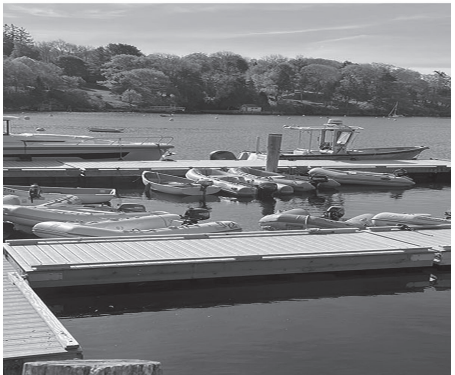
New Dingy Docks built by our Public Works Department.
