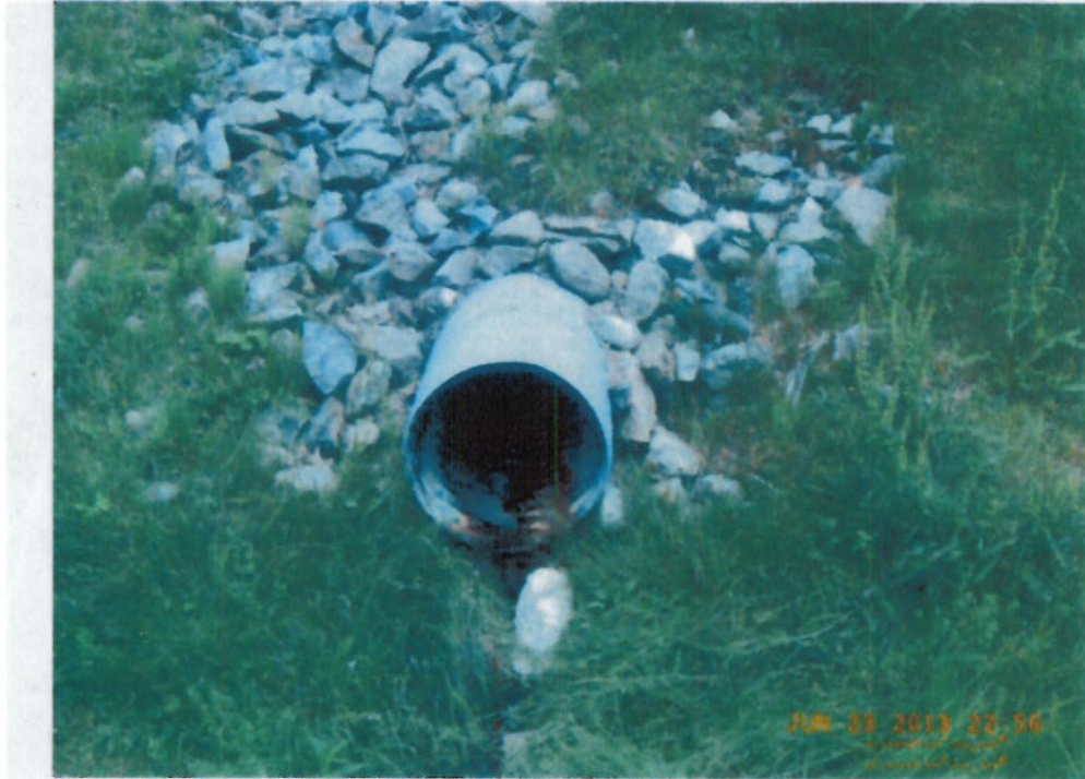
PA-3: Outfall which directs drainage from the west side of Pascal Ave. and to outfall PA-1.
