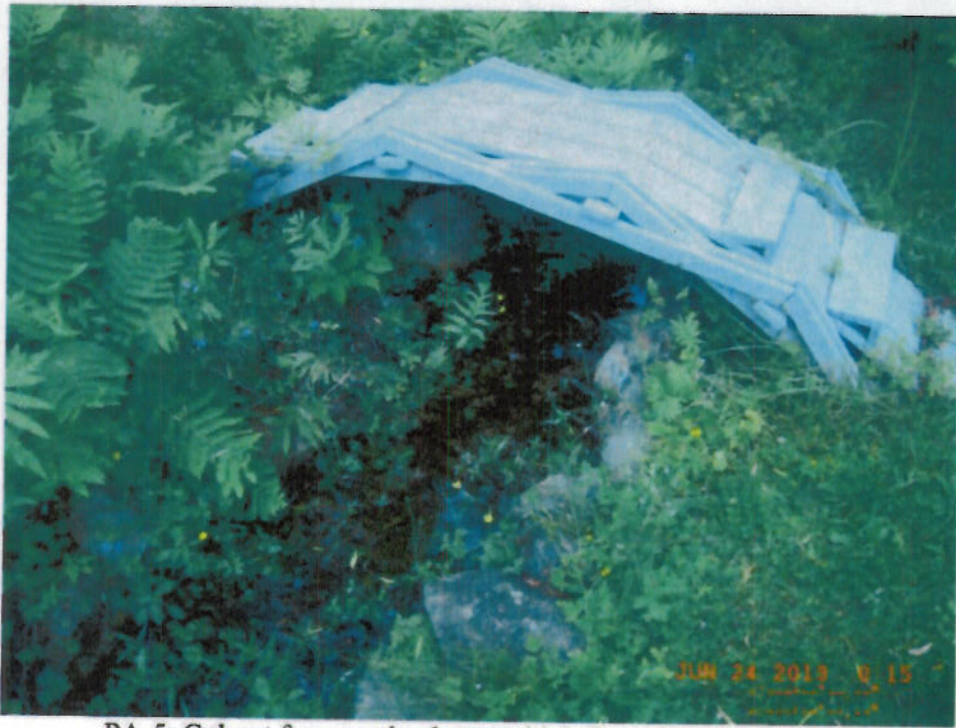
PA-5: Culvert from wetland area which flows towards PA-4B.
