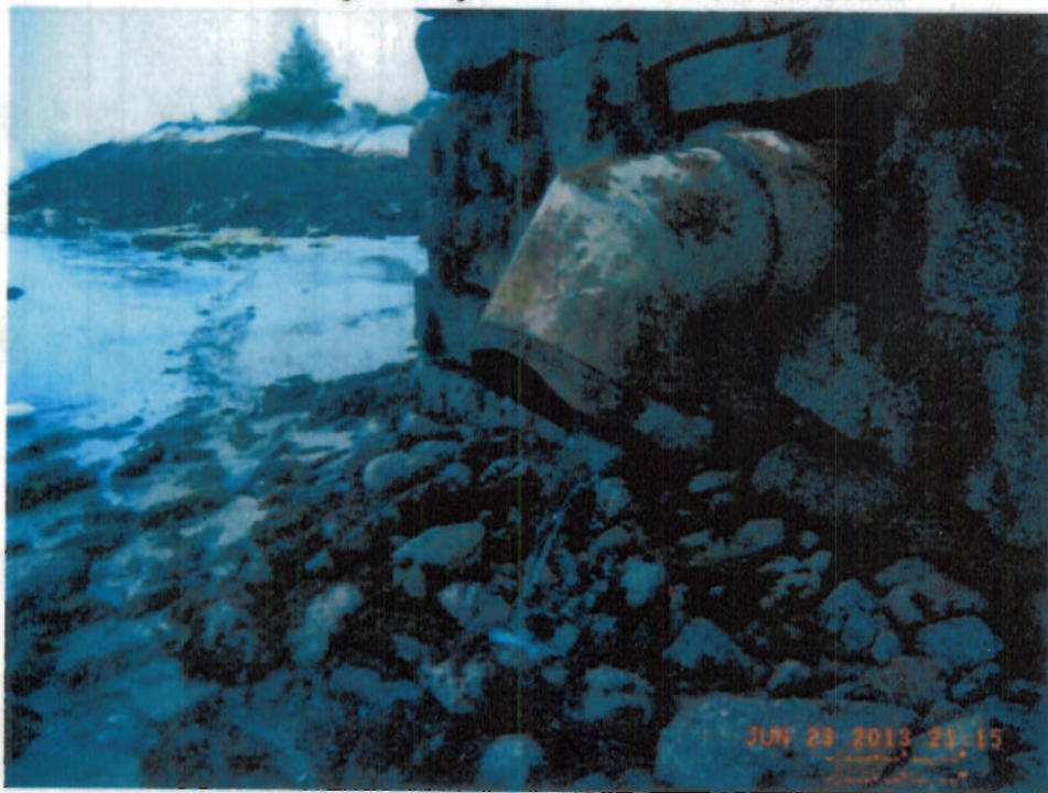
PA-1: Outfall located at Goodies Beach which discharges the Pascal Ave. drainage into Rockport Harbor.
